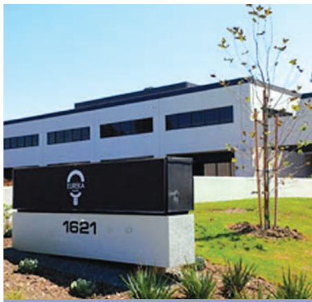
Project: The Eureka Bldg., Irvine
