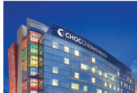
Project: Bill Holmes Tower @ CHOC Children's Hospital
