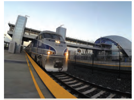
Project: Anaheim Regional Transportation Intermodal Center (ARTIC) Nominee(s): Clark Construction Group – CA, LP Dave Burrus Parsons Brinkerhoff Samuel Sims
