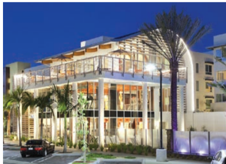
Project: Boardwalk by Windsor Nominee(s): TCA Architects Melissa Logan, Director of Marketing
