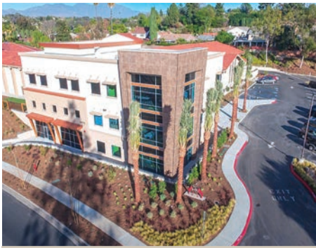
Project: Mount of Olives Children's Ministry Building Nominee(s): Mount of Olives Church Dave Scott, Manager Erickson Hall Construction, Inc. Jim Fisher, Project Manager
