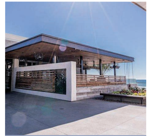
Project: Ola Mexican Kitchen Nominee(s): Ola Mexican Kitchen Anthony Andrews, Owner
