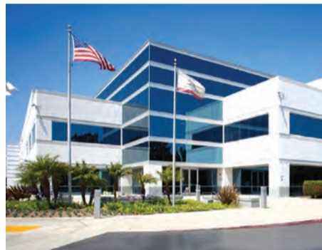
Project: Huntington Beach Distribution Center Nominee(s): Cushman & Wakefield Rick Ellison, Executive Managing Director Randy Ellison, Associate Director Kyle McGillen, Associate
