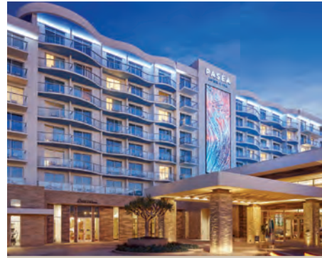
Project: Pasea Hotel & Spa Project Nominee(s): R.D. Olson Construction Matt Grubb, Vice President, Construction
