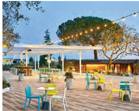
Project: Parasol Park Nominee(s): Slater Builders, Inc. Lizabeth Slater, CEO
