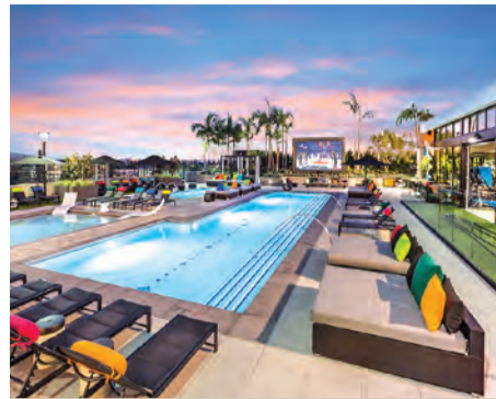
Project: The George Parking Structure and Amenity Deck Nominee(s): Slater Builders, Inc. Lizabeth Slater, CEO
