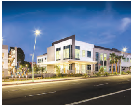
Project: Beach Boulevard Medical Pavilion Nominee(s): Oltmans Construction Company Anjana Bhowmik, Senior Project Manager Ware Malcomb Mila Volkova, Studio Manager Blue Sky HB Carol Ruggero, CFO
