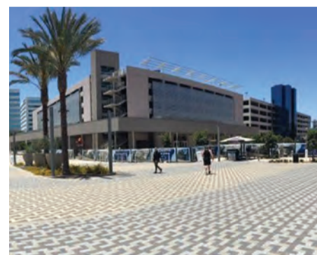
Project: Lakeshore Parking Structure Nominees: SENTRÉ Partners (client) John Brand, Chief Operating Officer Snyder Langston Richard Cavecche, Senior Vice President, Operations Alan Wardin, Senior Project Manager Erin Sommer, Assistant Project Manager Scott Hardy, Senior Superintendent Mark Lopez, Assistant Superintendent Kelsey Frazier, Project Engineer Gensler Thomas Ventura, Lead Architect
