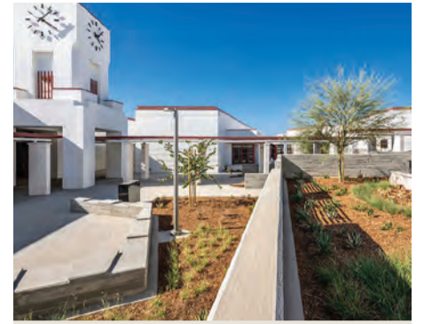
Project: Irvine Unified School District, Cadence Park K-8 School Nominee(s): C.W. Driver Jonathan Keene, Senior Project Manager PJHM Architects Kenneth Podany, CEO, Principal Architect
