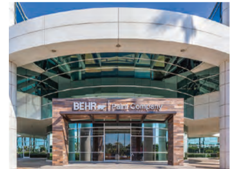
Project: Behr Paint Company Nominees: H. Hendy Associates Jennifer Bartelt, Project Manager Jeep Pringsulaka, Senior Designer DPR Construction Rudy Martinez, Project Manager
